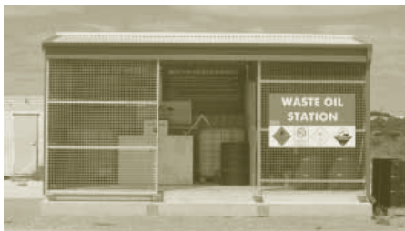
Tailem Bend waste oil collection facility in South Australia.
