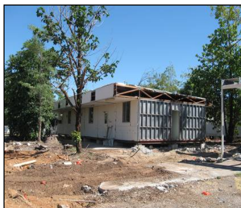
Figure 6.2 Building 20 at JFS ready for relocation
