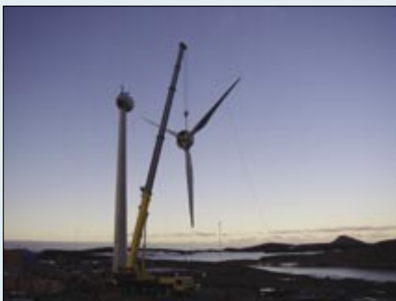
Installing the blades.
