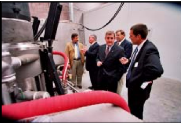
The Hon Mr. Ian Macfarlane, Senator John Tierney The Hon Mr. Bob Baldwin, Mr. Russ Teall & Mr. Andrew Hill Inspect internal workings of the plant. 12 th March 2003
