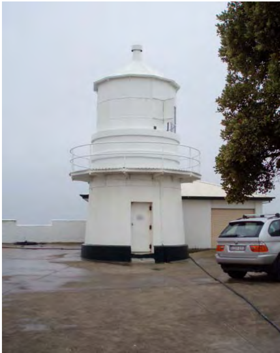
Figure 4: Nobby's Lighthouse (view from west), with garage visible at right and parapet in the background.
