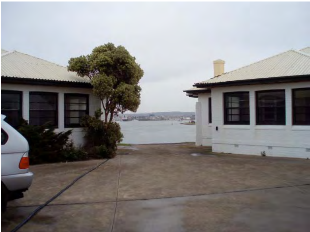
Figure 6: View from the base of Nobby's Lighthouse through the two keepers' cottages toward the port of Newcastle.
