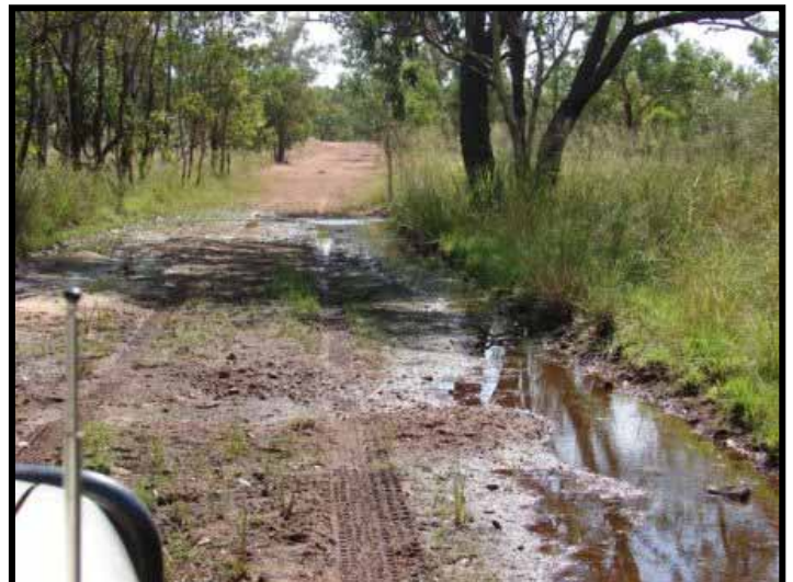
Image 3 – Water over the road to Maguk To avoid long term damage to tracks, some areas need to dry out before they are suitable for traffic.
