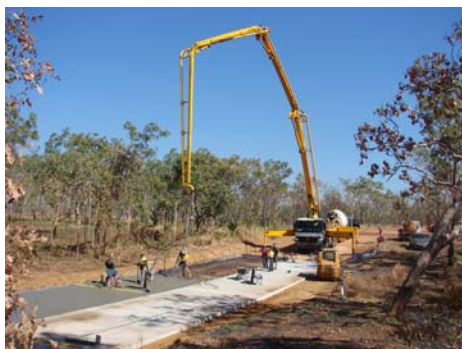
Workers concreting floodway section on the Jim Jim Falls road.
