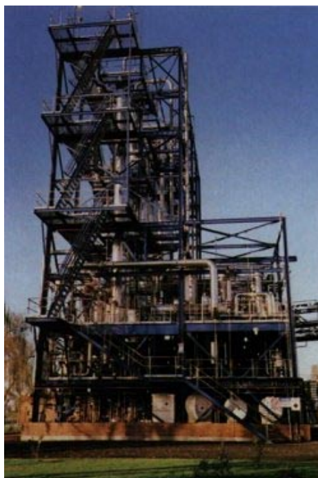
Figure 6.1 The ethanol plant at Manildra's Bomaderry plant near Nowra. ( http://www.manildra.com.au/prospectus/prospectus6.html )
