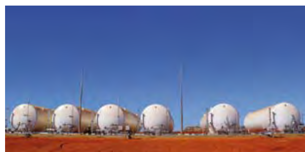
Broome Fuel Storage Facility
