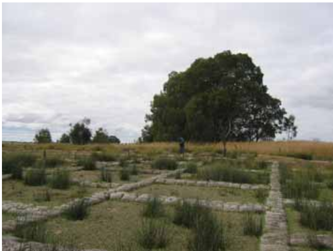
New protection works layout, east toe of Snake Island, July 2005 (JL)
