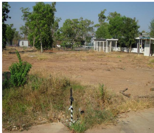
Figure 6.2 JFS site following demolition and removal of buildings
