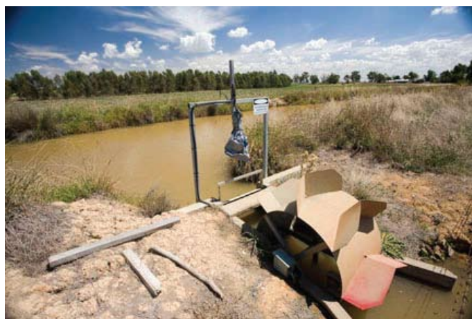
Goulburn-Murray irrigation canal (J Baker)
