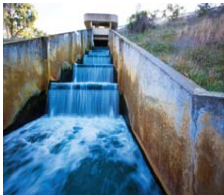
Molongolo Water Quality Control Centre (D. Markovic)
