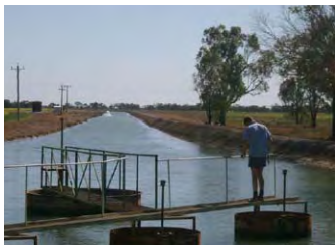
An on-farm channel at a corporate farm near Hay, NSW. The channel is used for delivering groundwater, and for delivering water that the farm pumps from the Lachlan River. Photo: M.Chapman
