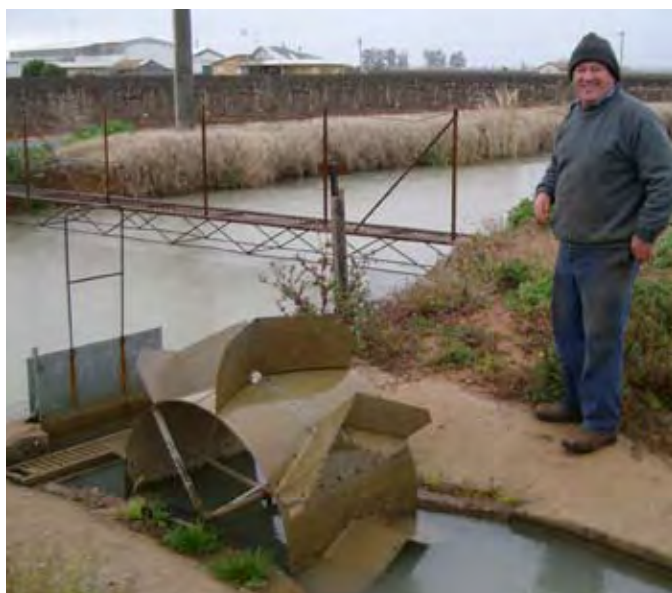
Dethridge wheel metering the water taken off the water authority channel and on to the farm. Photo: L. Chapman
