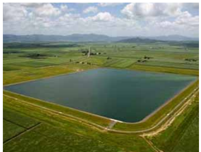
One of the Project's recycled water irrigation dams (Photo: Mackay Regional Council)
