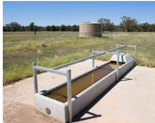
Bore stock water points at a property near Boomi in northern NSW have replaced open bore water channels, reducing evaporative losses. (A Mostead & DEWHA)
